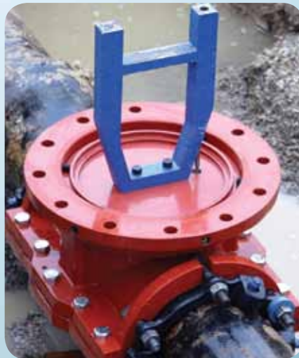
Internal equalization completion plug installed.
